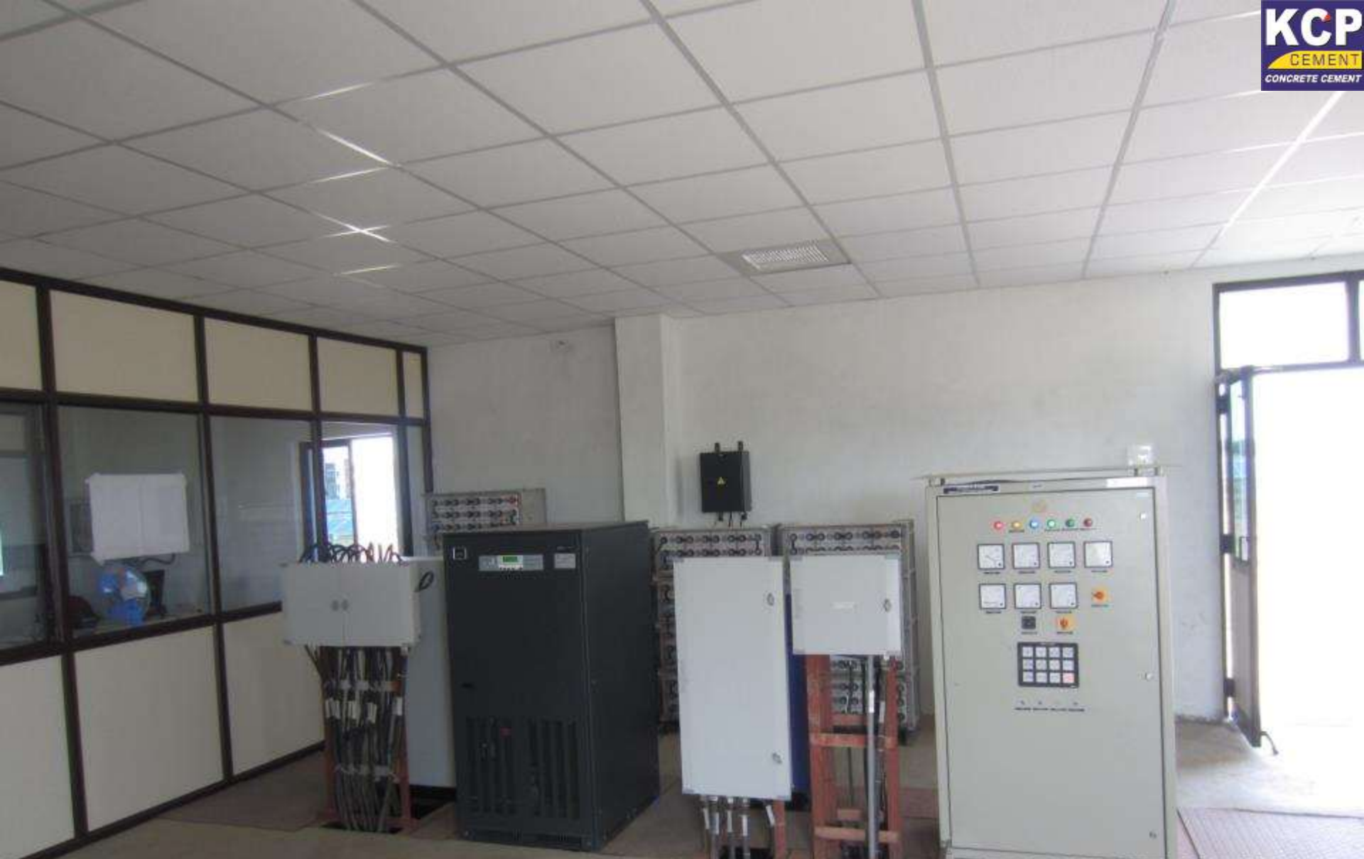
UPS AND BATTERY CHARGER
